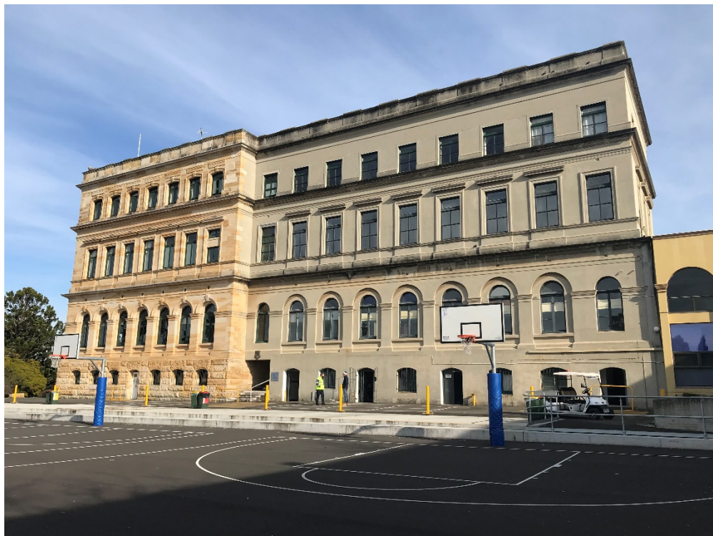
Figure 6 - View towards the eastern facade of the Main Building (left of image) and the Doyle Wing (right of image) from the basketball courts located within the Third Yard.
