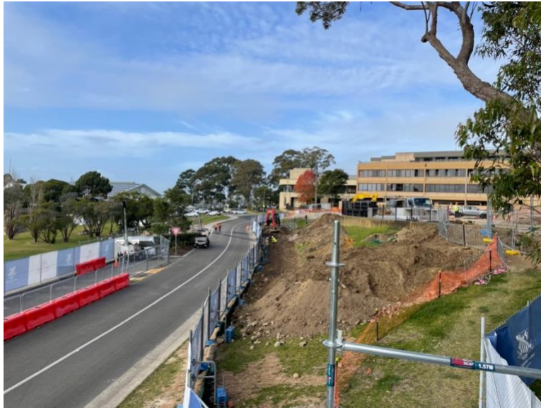
Figure 3 Site view from elevated access walkway - boundary and sediment fences.
