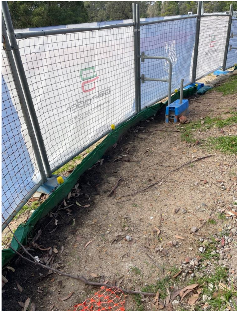
Figure 4 Boundary sediment fences
