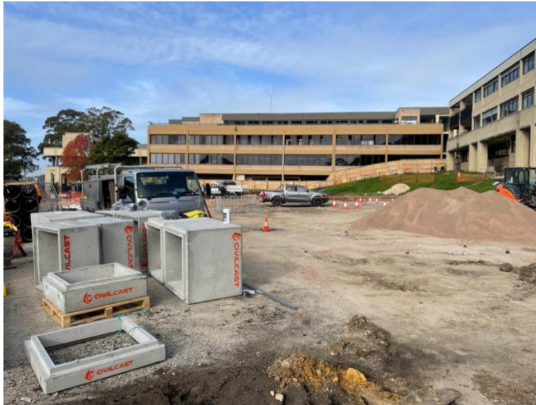
Figure 9 Upper terrace, laydown area.
