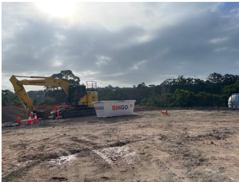
Figure 6 Construction general waste bins in place
