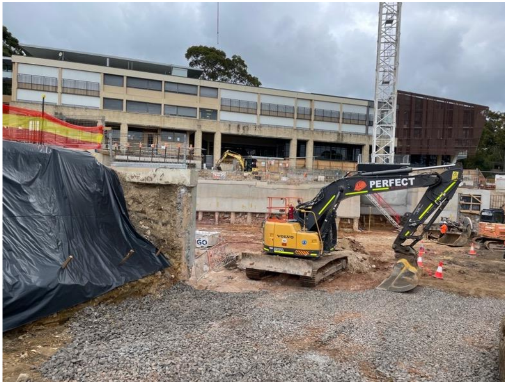
Figure 4 Boundary sediment fences in place and functioning correctly
