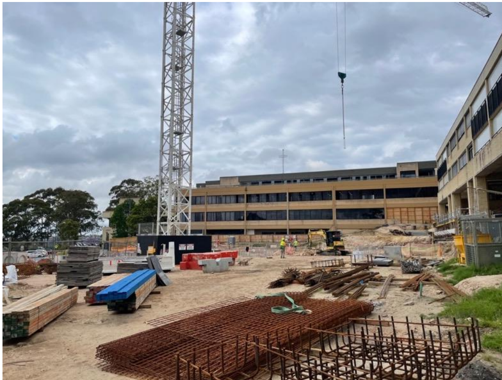
Figure 9 Upper terrace, laydown area
