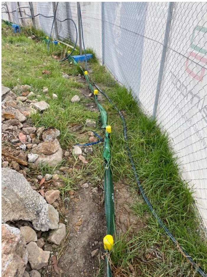
Figure 4 Boundary sediment fences in place and functioning correctly
